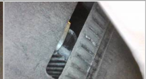
Finally, the belt with 10 ft/lb applied using the belt tensioning tool 3)
